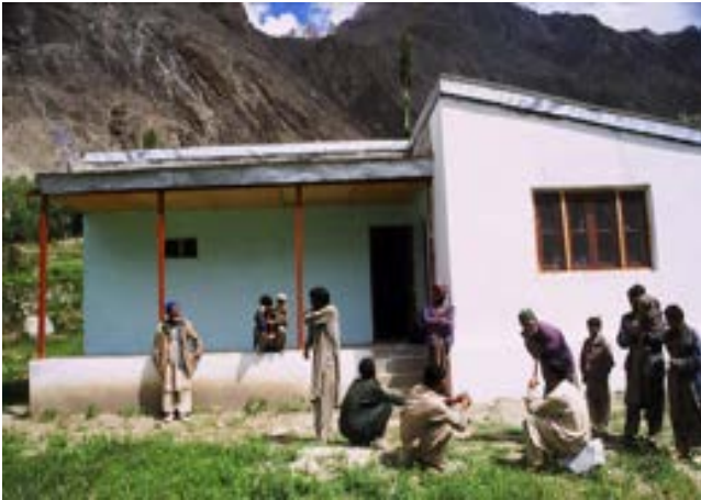
Krankenstation in Thongal
